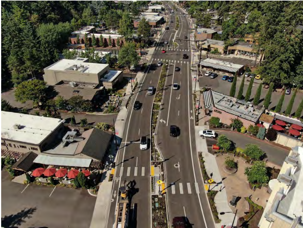
Example of arterial-scale streetscape improvements similar to those possible on Highway 20, showing new sidewalks, lighting, bike lanes, mid-block crossings and median landscape (Boones Ferry Road, Lake Oswego, OR)
