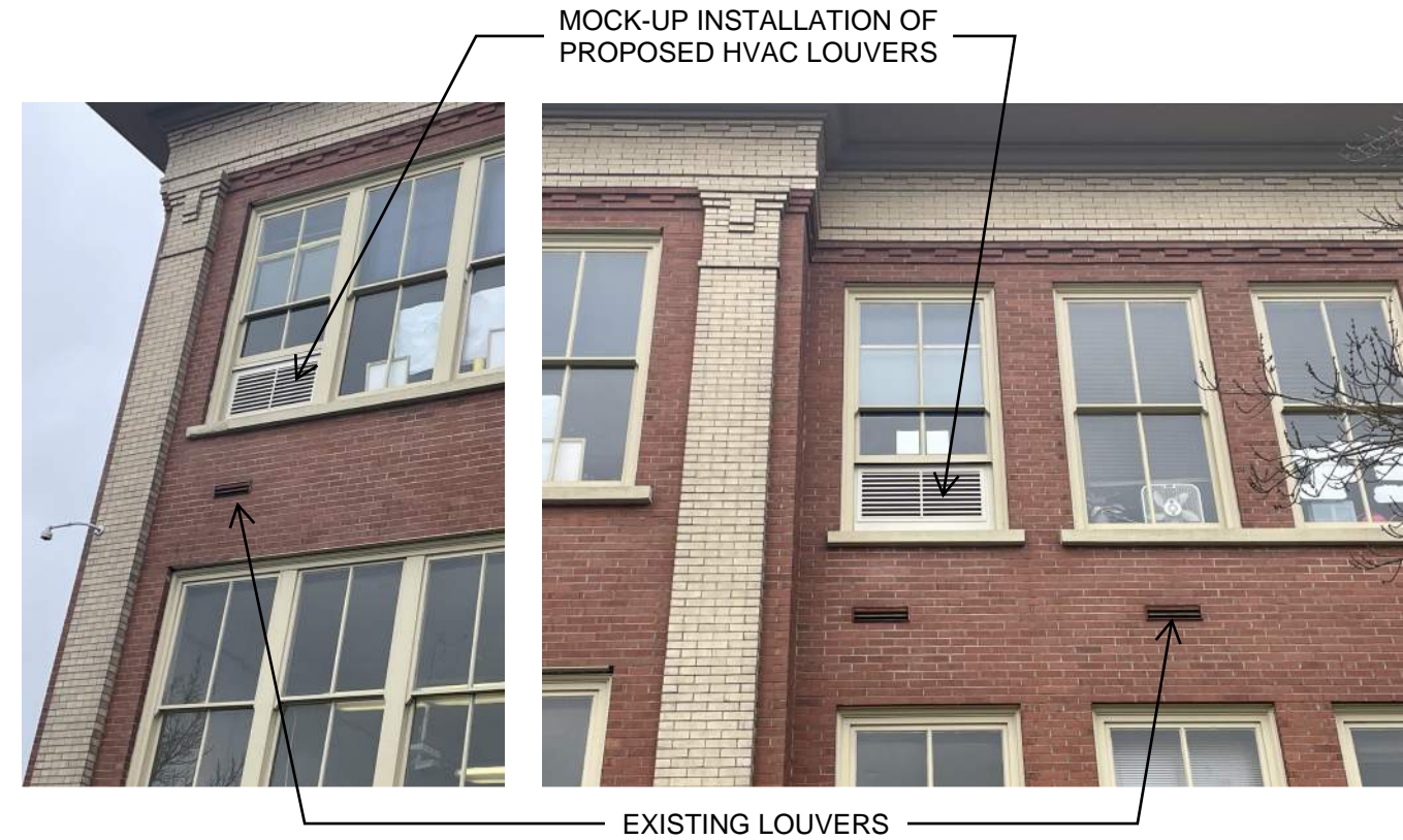
4 ENLARGED WINDOW ELEVATION, TYPICAL
