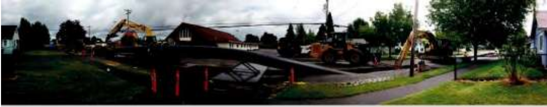
Water line construction on Hill Street.
