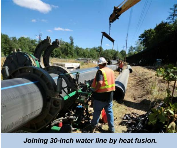
*Joining 30-inch water line by heat fusion.*
