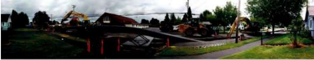
Water line construction on Hill Street.
