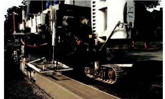
Curb installation for the Oak Street construction project.
