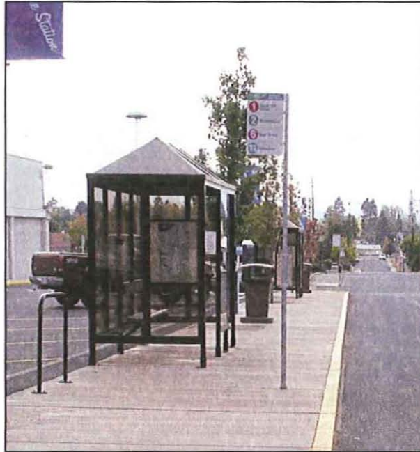
Exhibit 10-3 Bend Bus Shelter with Route and System Information
