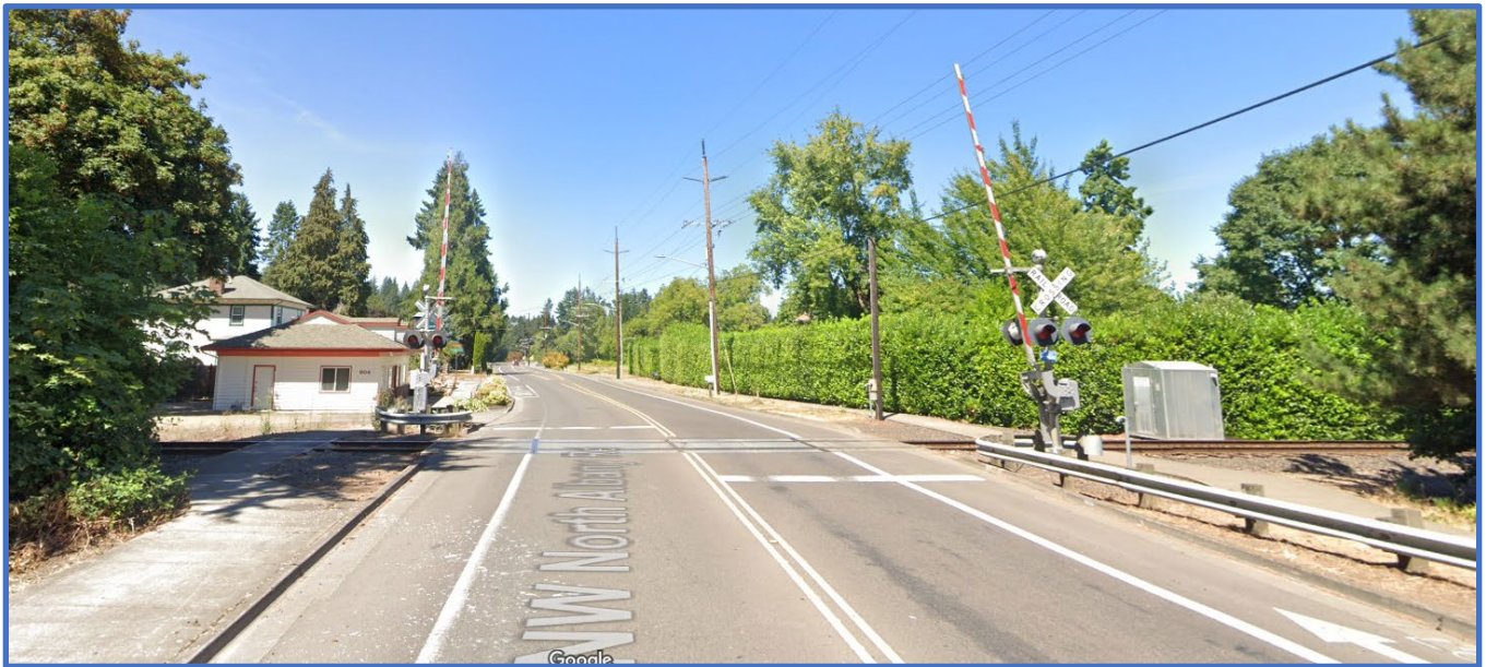
Figure 2. At-Grade Rail Crossing at North Albany Road
